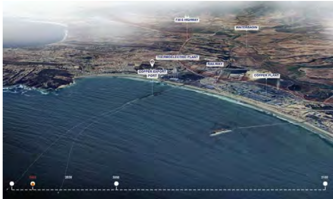
04 | Landscape's Current Condition
