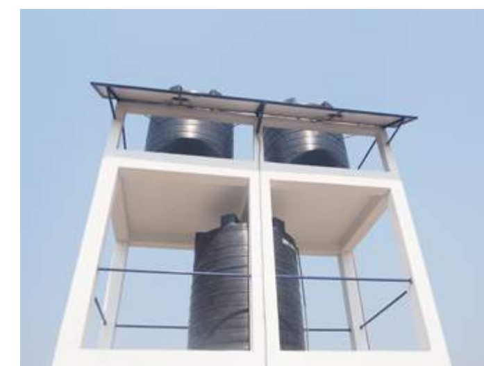
Solar power and storage for irrigation well
