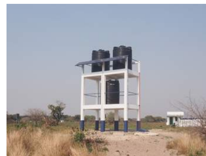
Solar power and storage for irrigation well
