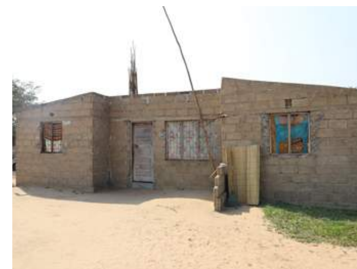
Local housing constructed with cement (limestone and clay), water, and sand from rivers
