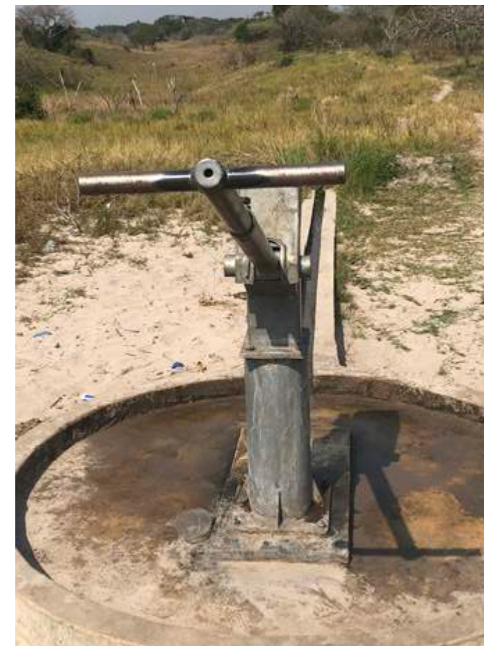
Manual hand pump for irrigation well
