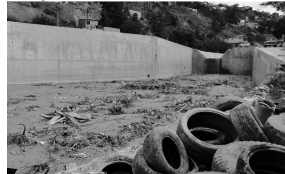
01. Concretized channel: Disconnecting the natural flow of water and life.
